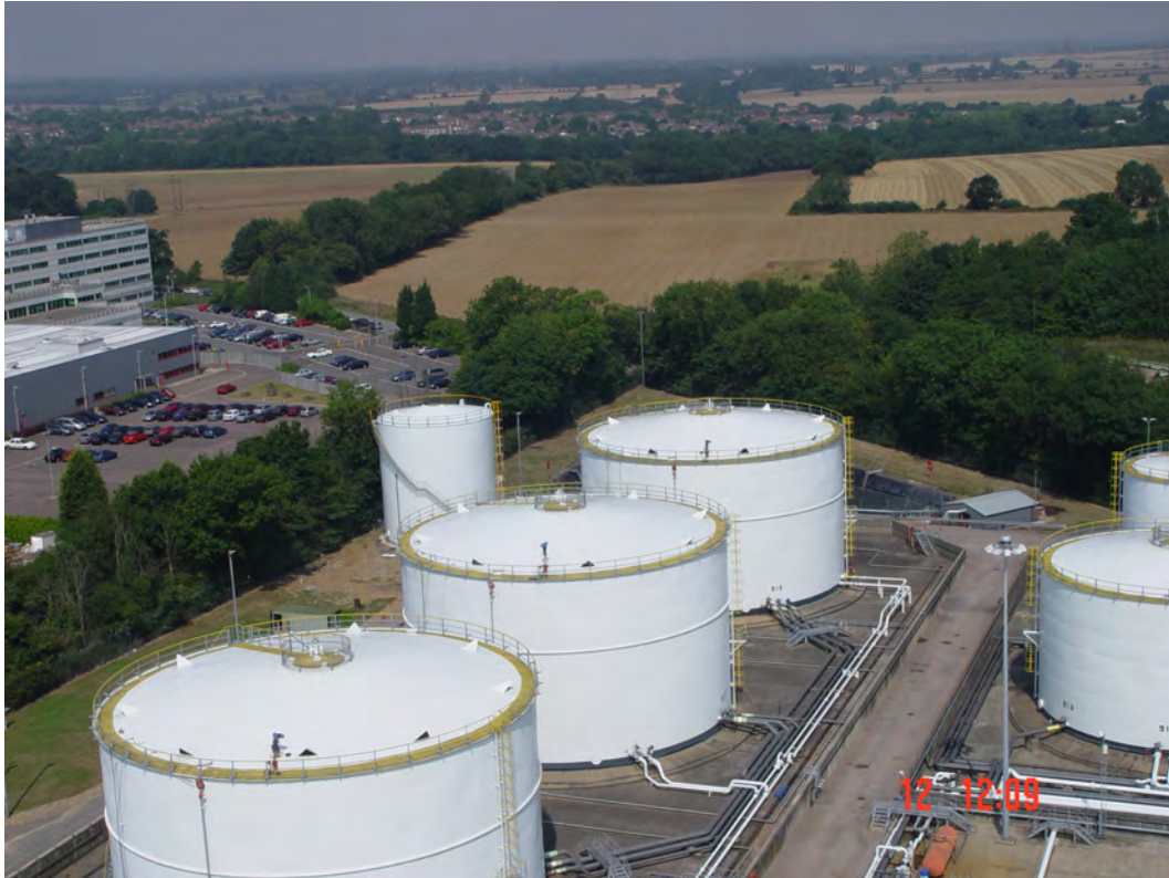
Figure 2 Pre-accident view of Buncefield Oil Storage Depot
