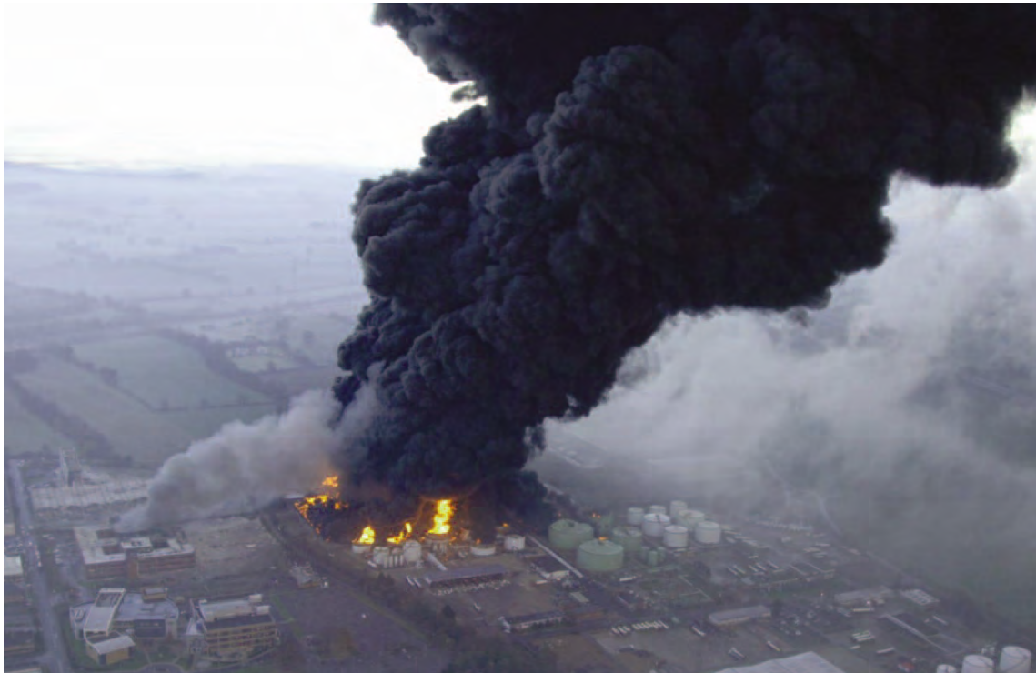
Figure 1 Ensuing fire at the 2005 Buncefield oil and gasoline terminal explosion
